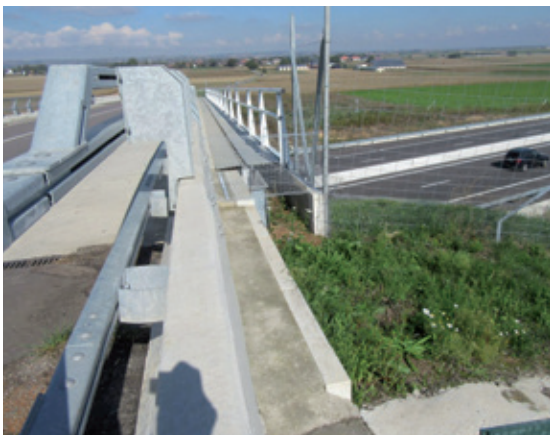
Figure 44: © VINCI Autoroutes Photo Library
