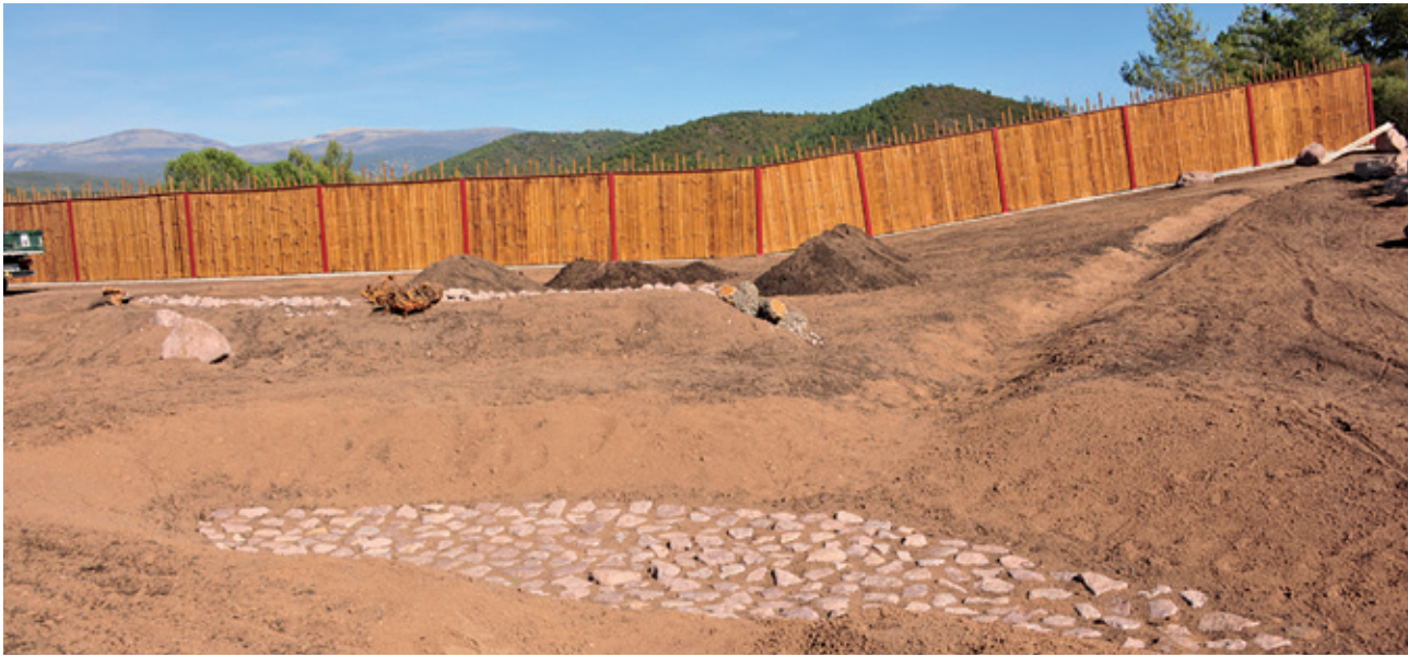
Figure 22: In the dry Mediterranean context, creation of ditches to feed the ponds. ©M. MARTINI.
