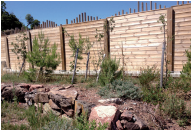
Figure 27: Eco-terrace deliberately collapsed to reach soil level. © VINCI Autoroutes photo library.
