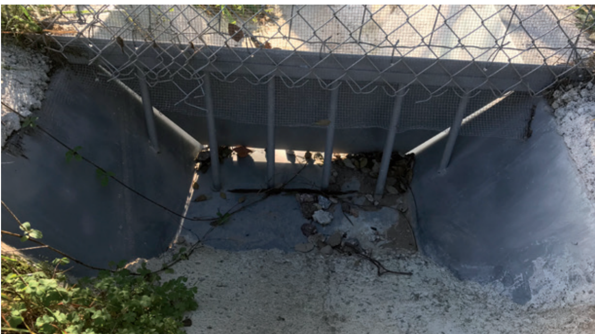
Figure 18: SANIEZ prototype stainless steel ditch module to secure the ditches by replacing conventional concrete sills. ©Cabinet X-AEQUO.
