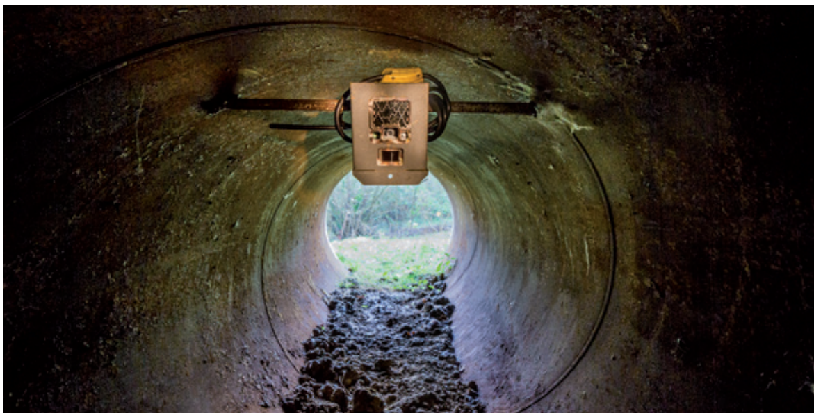
Figure 53: Camera trap set up in a 120 cm eco-duct. ©Alexis Orseau/LPO France.
