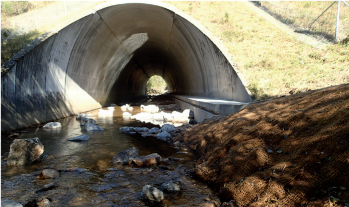
Figure 86: General view of the Deiro structure and its re-adaptation for small fauna (photos taken in the worksite phase). ©GREGE.
