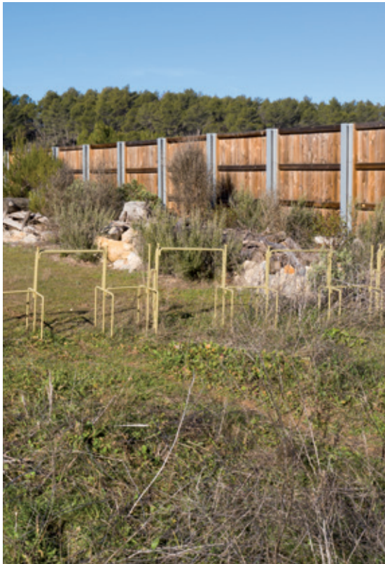
Figure 32: Anti-intrusion barriers. ©VINCI Autoroutes.
