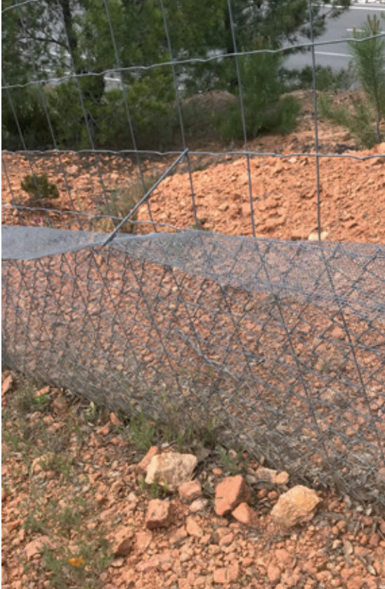
Figure 17: Fine mesh liner fitted to a fence for small fauna. The most successful arrangement has a tensioning wire attached to angle irons. ©Cabinet X-AEQUO.
