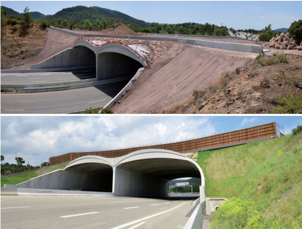
Figure 21: Revegetation by seeding the slopes of double-arch bridges prevents gullying. ©M. MARTINI.
