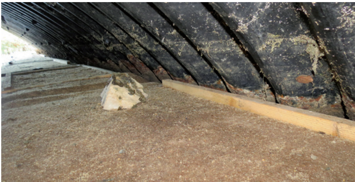
Figure 81 : Marking relief (stone) widely used by wildlife, positioned on the floating pontoon of a hydraulic road structure. ©LPO France.
