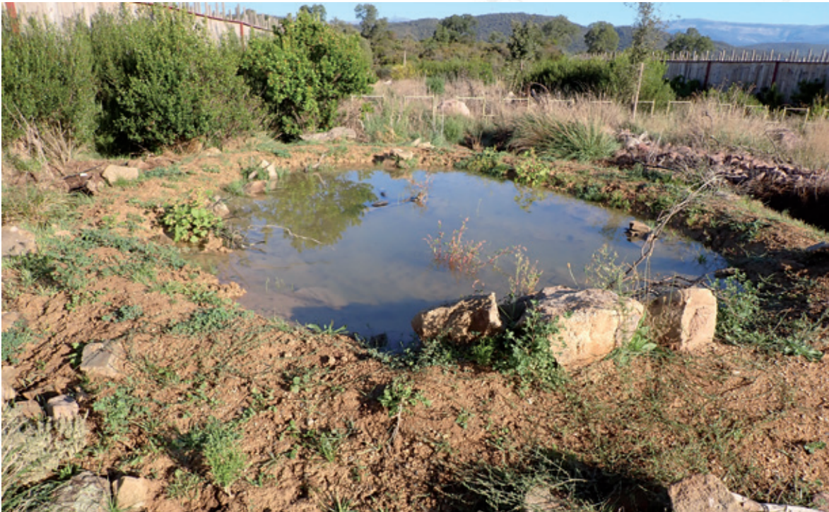
Figure 25: Testing of protection using a buried sheet of mesh (Adrets-de-l'Estérel eco-bridge). The alternation of sand, geotextiles, membranes (Bidim/EPDM) combined with a mesh grid with anchored plating irons gives good results after one year. ©Cabinet X-AEQUO.
