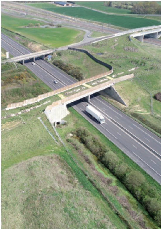
Figure 47: Bas-Bry Eco-bridge, a crossing for wildlife above two infrastructures. ©VINCI Construction Terrassement. ©VINCI Construction Terrassement.
