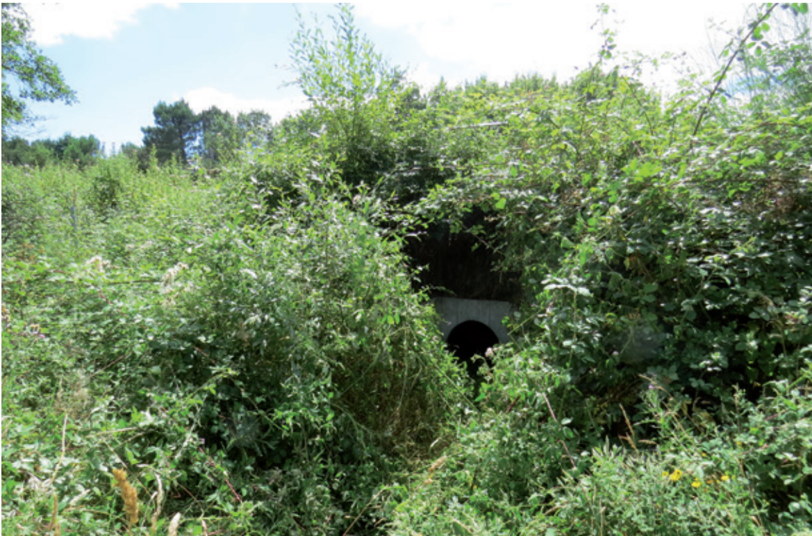
Figure 58: Entrance of an 80 centimetre in diameter eco-duct overgrown with vegetation making monitoring the entrance by camera trap impossible. ©ASF/LPO France.
