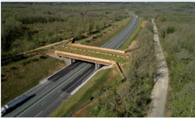
Figure 6: Le Causse Eco-bridge - Les Grands Genèvevriers A89. ©KOOX.
