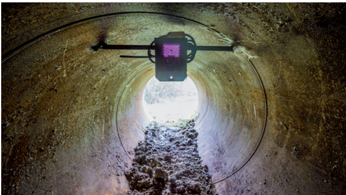
Figure 35: Example of a clayey substrate with dry clods in a 120-centimetre-diameter eco-duct. ©Alexis Orseau/LPO France.
