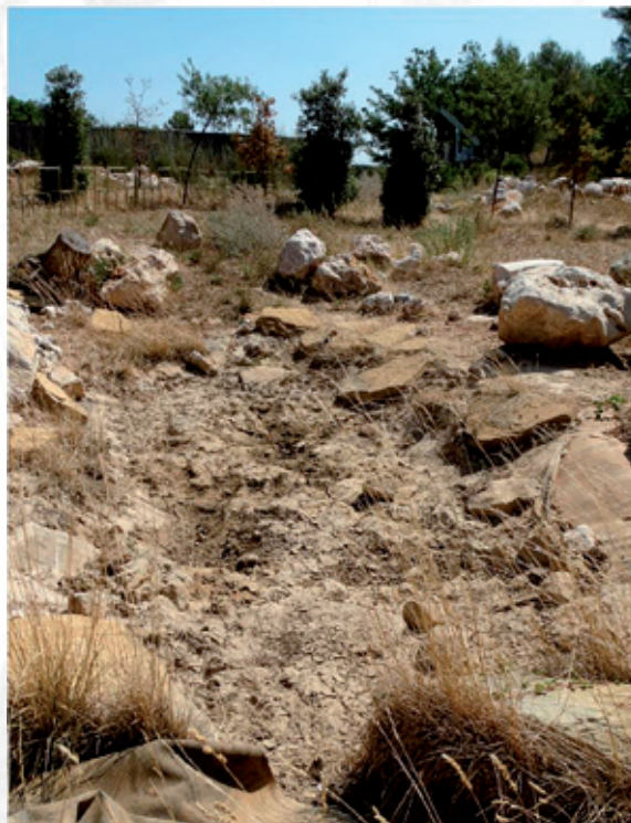
Figure 26: A pond trampled by wild boar. Due consideration needs to be made when creating the pond to ensure its durability and the efficacy of the seal. ©VINCI Autoroutes.
