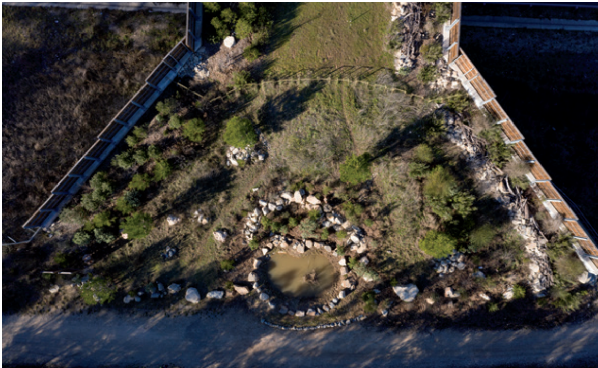
Figure 24: Rockfill around the pond to protect it from wild boar. © VINCI Autoroutes photo library.
