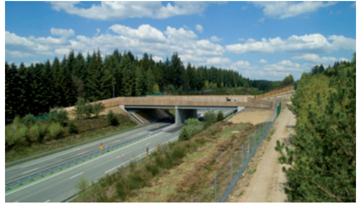
Figure 5: La Pologne A89 Eco-bridge. ©KOOX.
