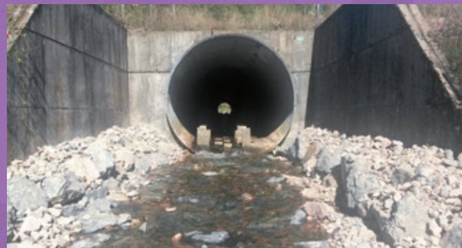
Figure 39: Before/After: The stilling basin has been filled in, the 40-centimetre fall at the exit of the culvert removed and rough elements added inside the culvert to influence the flow speed. ©VINCI Autoroutes Photo Library
