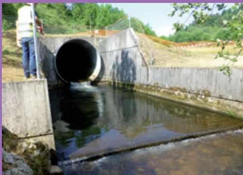
Figure 39: Before/After: The stilling basin has been filled in, the 40-centimetre fall at the exit of the culvert removed and rough elements added inside the culvert to influence the flow speed. ©VINCI Autoroutes Photo Library
