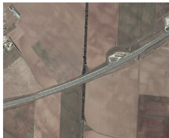
Figure 65: Example A83 (Deux-Sèvres) intersecting an obvious ecological corridor (wooded former railway) in the middle of an intensive agricultural landscape. ©IGN, 2002.
