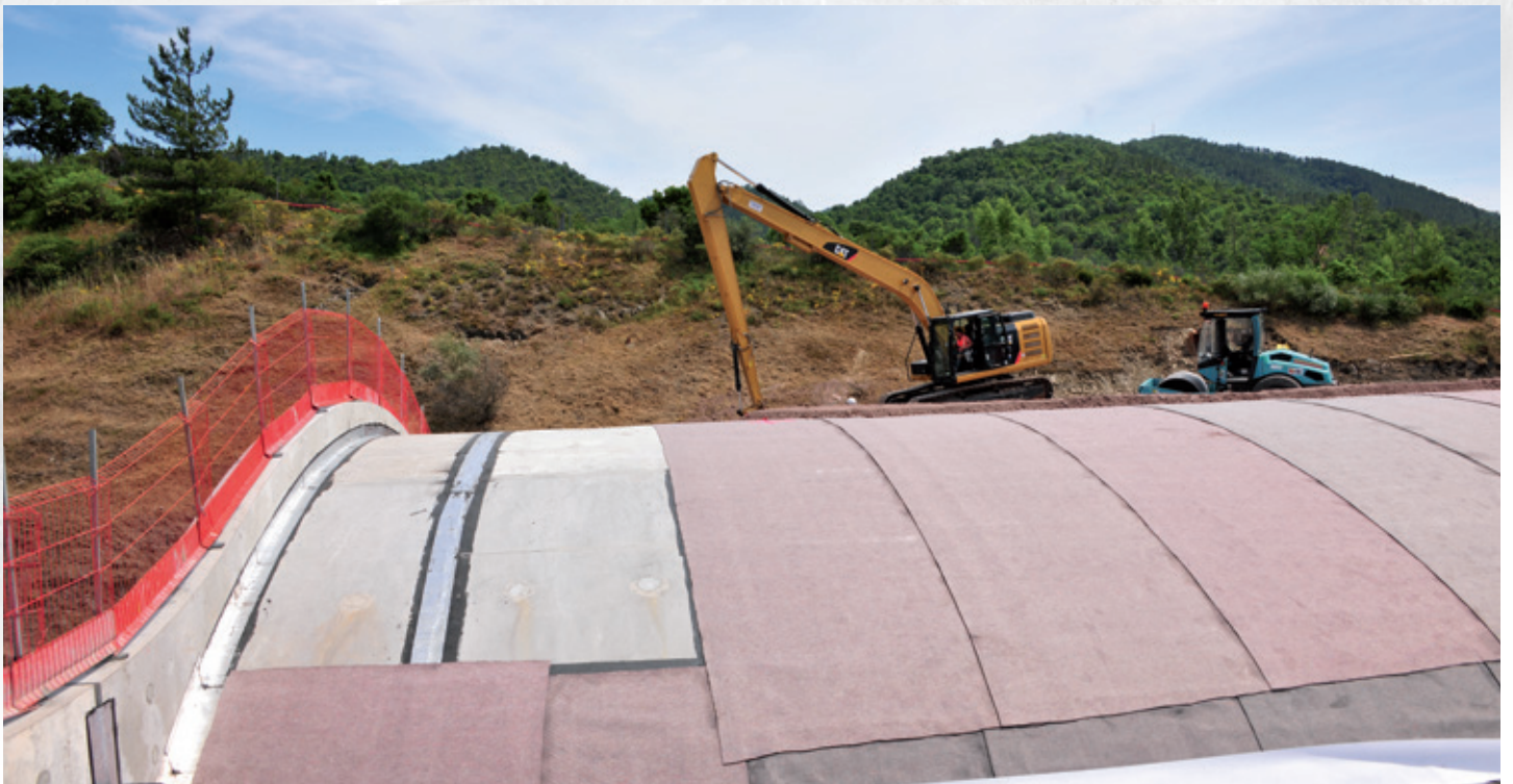
Figure 11: Deck of an eco-bridge before being covered by material. ©M. MARTINI.
