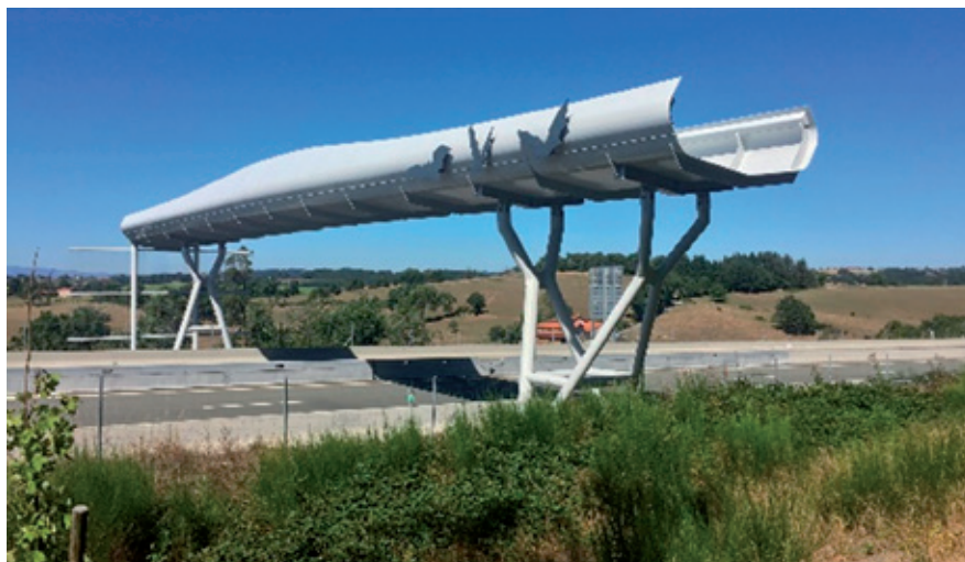
Figure 85: Bat-bridge (cradle structure) at Moulin-Paris on the A89.
