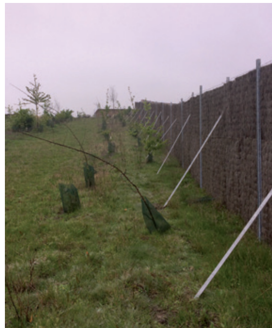
Figure 16: When using heather for visual barriers, reinforce the fence with struts at regular intervals (every second fence post). ©VINCI Autoroutes.
